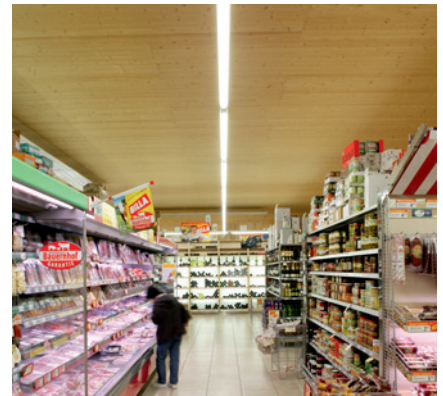
Trunking systems and batten luminaires
